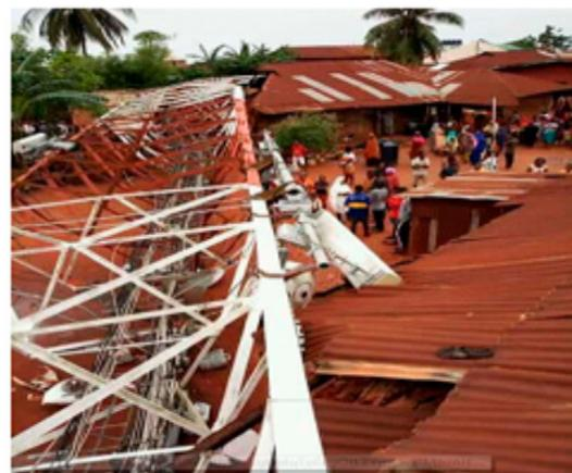
**Figure 4.** Fallen telecommunication mast and damage to buildings.
