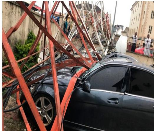
**Figure 3.** Fallen telecommunication mast and damage to cars.
