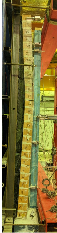
Figure 9: Deflected Shape of the Wall After Veneer Cracking
